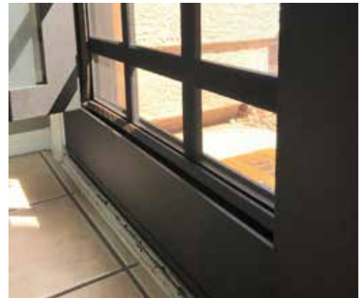
Fiberglass insect screen to keep out the critters when using operable glass to ventilate.
